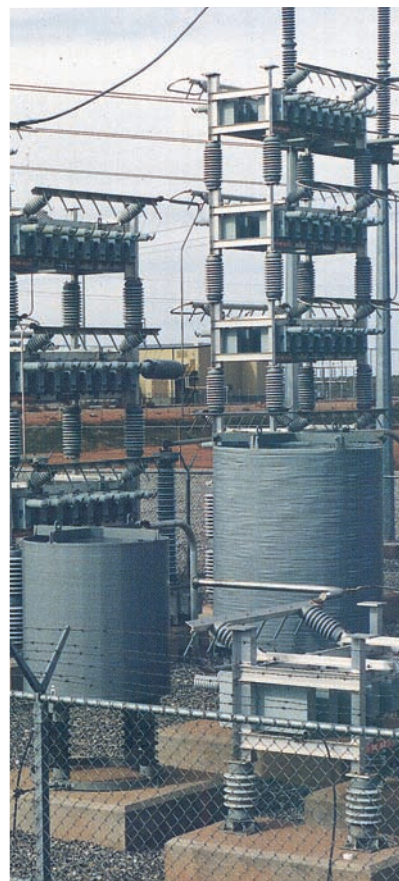
Fig. 8 Filter reactors
