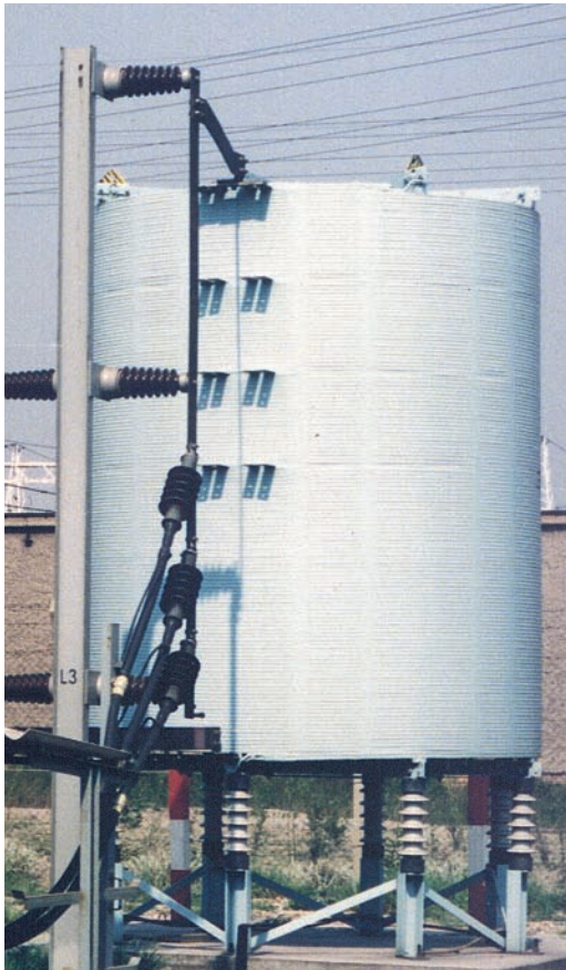
Fig. 5 Buffer reactor for E.A.F.
