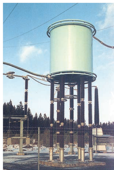
Fig. 17 HVDC-Smoothing reactor
