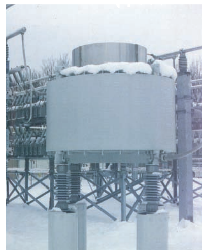
Fig. 9 Filter reactors with de Q'ing rings
