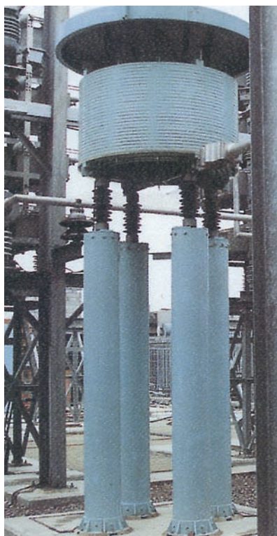
Fig. 36 Filter reactor with top-hat and pedestal
