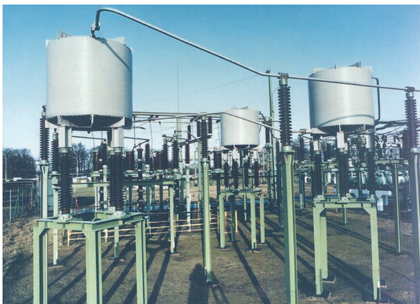
Fig. 3 Single phase series reactors
