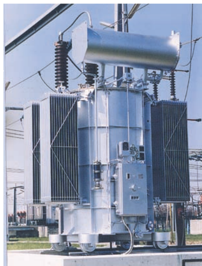
Fig. 27 Arc suppression coil 110 kV
