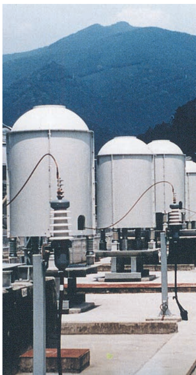
Fig. 35 Filter reactor with sound shield
